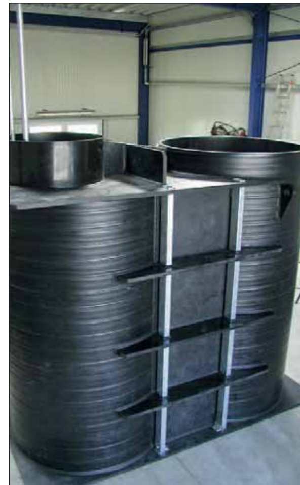
1-fold lysimeter station for Slovakia under construction
