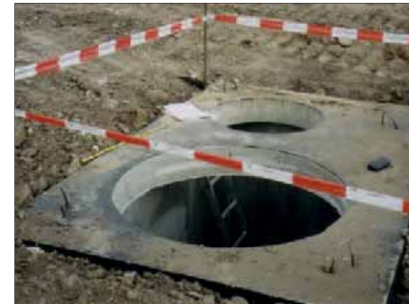
Top panel of a containerized concrete lysimeter
