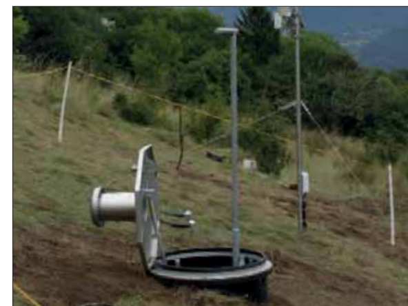
Access shaft of the lysimeter station
