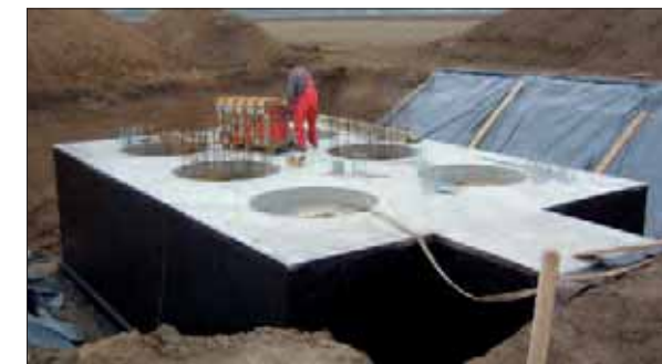
Preparation for the installation of the lysimeter collar
