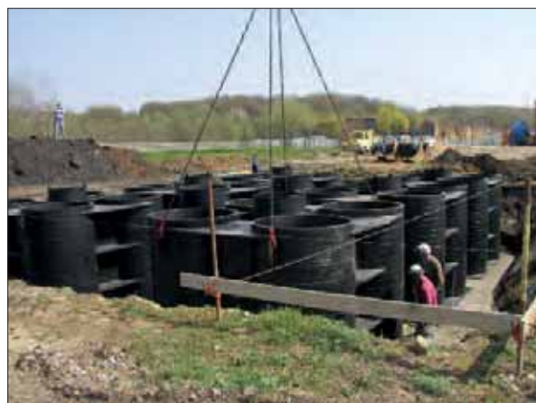
Lysimeter station under construction
