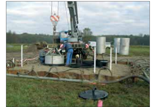
Insertion of the lysimeters into the station
