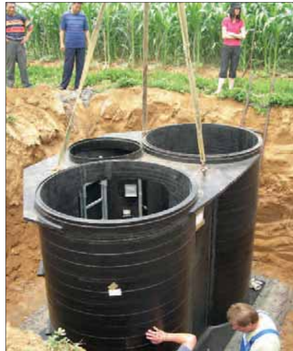
Installation of the 2-fold lysimeter station
