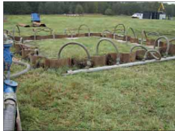
Area of the steel piling (5 m x 6 m) with groundwater lowering
