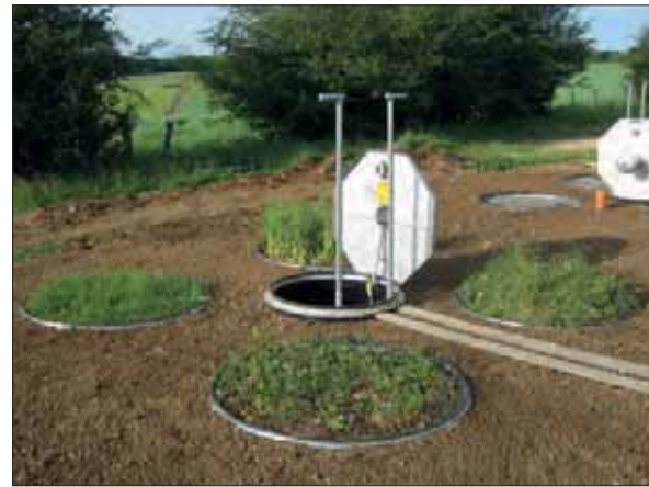
Lysimeters with vegetation shortly after installation
