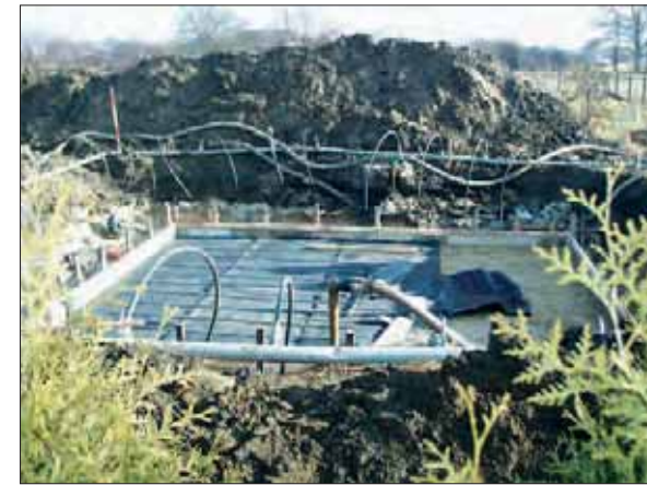
Construction of the lysimeter stack
