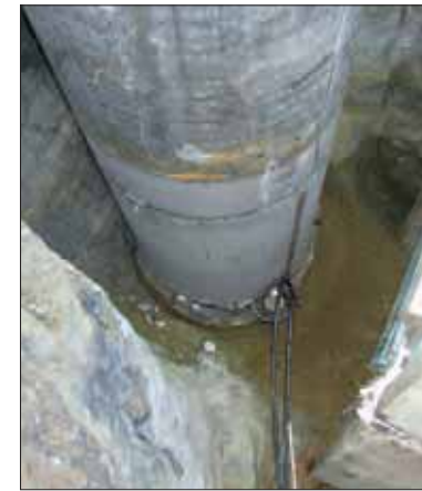
Monolith excavation in 4 m depth
