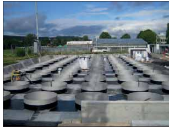
Lysimeter station under construction
