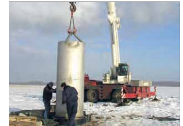
Insertion of the lysimeter in the station
