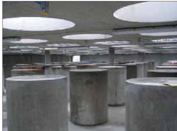
Construction of the basement for the lysimeter station
