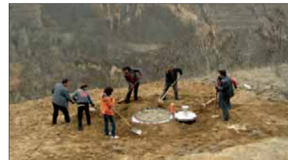
Installation of a lysimeter without heavy equipment
