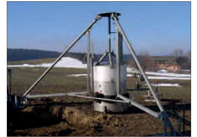
Excavation Technology for a 1 m 2 soil monolith
