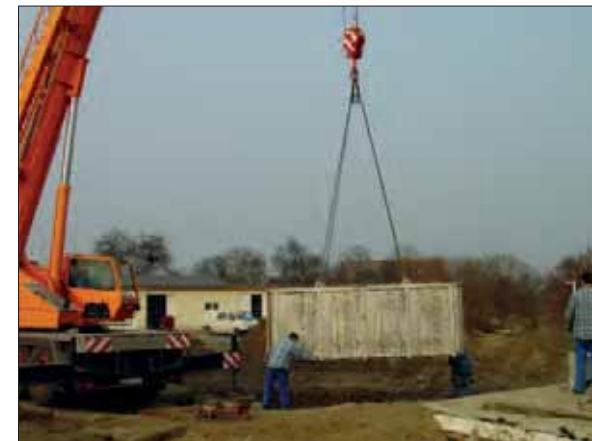
Putting the filled lysimeter vessel in its place
