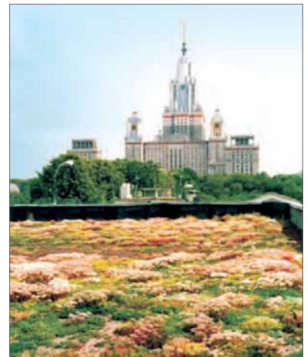
Pilot green roof Lomonossov University Moscow
