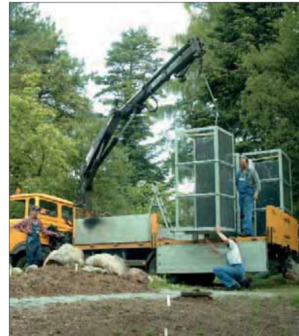
Installation of the root boxes in the Root Stack
