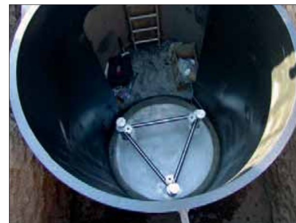
Load triangle for weighing system
