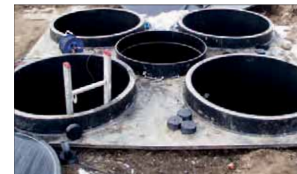
Installation of a 4-fold gas migration simulator station
