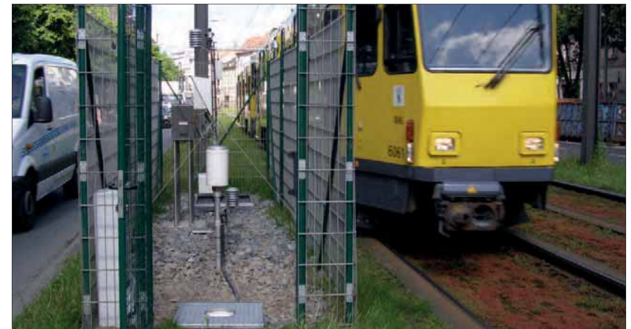
Urban track bed greening with embedded platy lysimeter and meteorological measuring station
