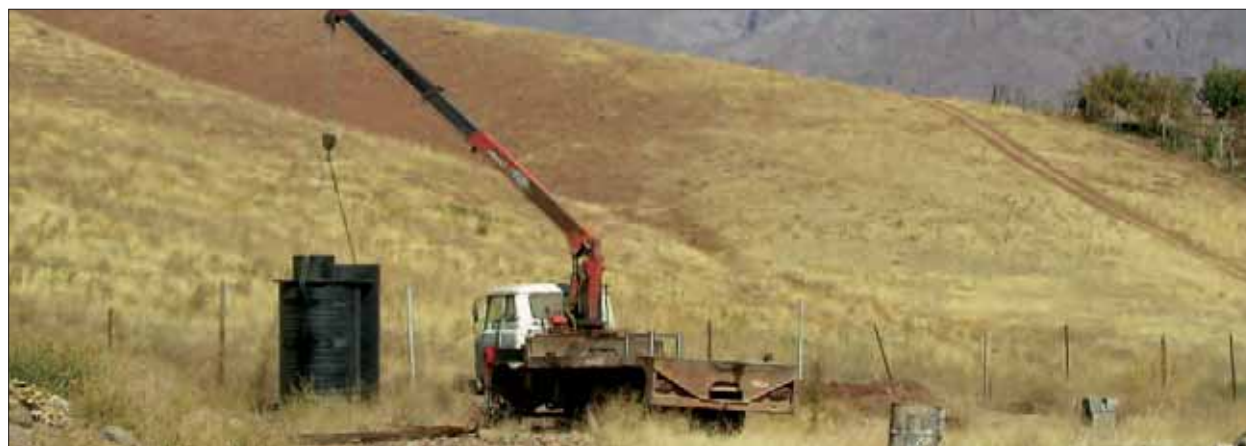
Installation of the PE-HD lysimeter station
