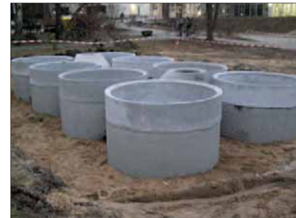
None containerized concrete lysimeters under construction
