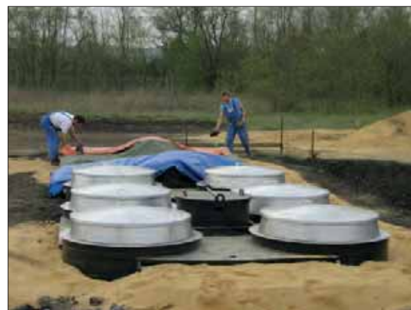
Lysimeter station at Homécourt shortly after finishing the construction works
