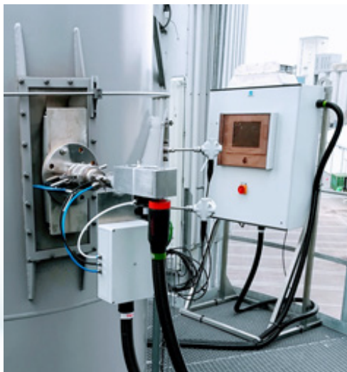
AMESA-B Control cabinet with sampling probe
